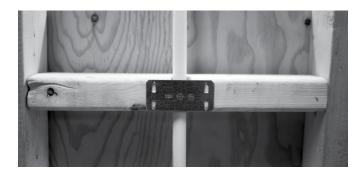
Protect pipe from nail damage where appropriate.
