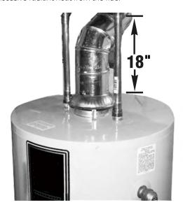
SuperPEX can be piped directly to the heater tapping on an electric hot water heater using metallic termination fittings.
