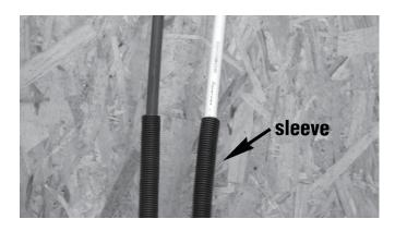
Protect pipe with non-metallic sleeves where it penetrates a slab or foundation.
