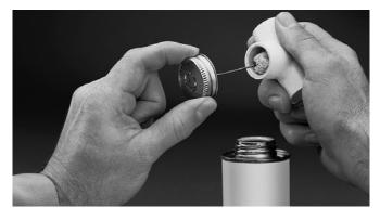
**4.** Using a dauber or natural bristle paint brush, apply solvent cement liberally on the pipe and sparingly in the fitting socket. Apply only CPVC cement conforming to CSA B137.6 and ASTM F493.
